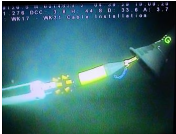
Figure 10.3-14: Inter-Array cable (with cable protection system) being pulled into a foundation.
