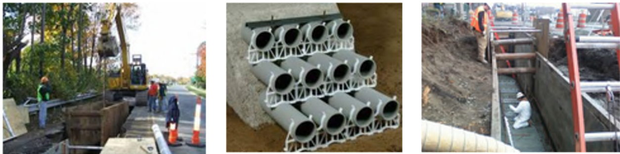
Figure 10.3-19: Onshore open trench and duct bank.
